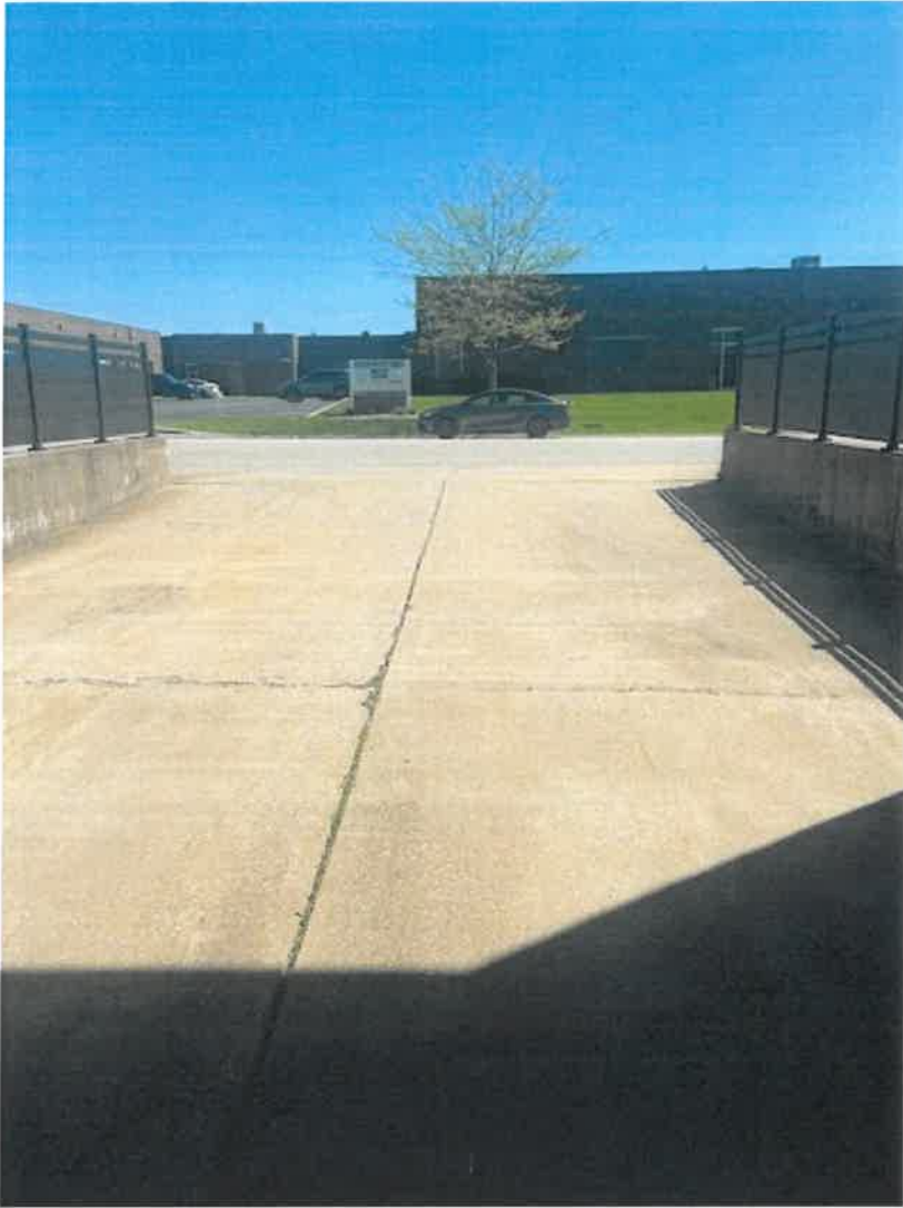
Sewer access just to right of Car
